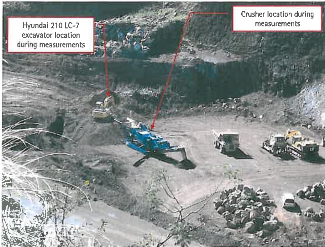
Photo 3 – View of Excavator & Crusher Operating
